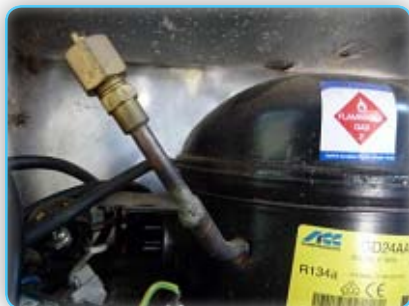
Process tube with Schrader valve
