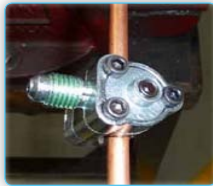
Bullet piercing valve disassembled (left) and assembled on pipe (right)
